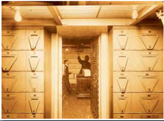
Within its vaults, the OCC held the U.S. government bonds that secured national currency.
