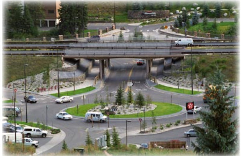
Figure 4: Roundabouts at an Interchange (Vail, Colorado)
