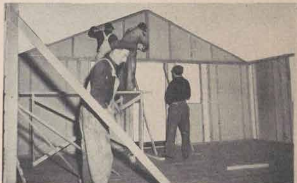
Figure 19. Erection and bolting of gable end.
