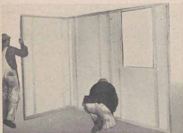
Figure 15. Erecting three corner panels.
