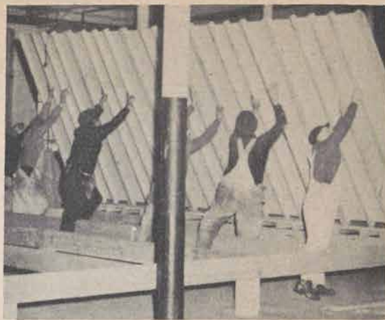
Figure 10. Lowering assembled floor section.
