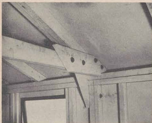
① Figure 28. Detail of connections at T-1, T-4 and T-5. ②
