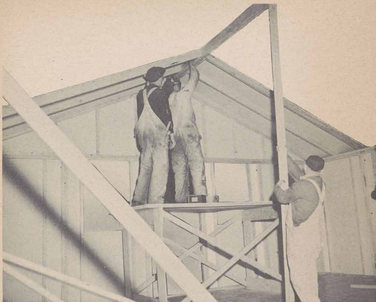
Figure 25. Erection of first two roof panels.
