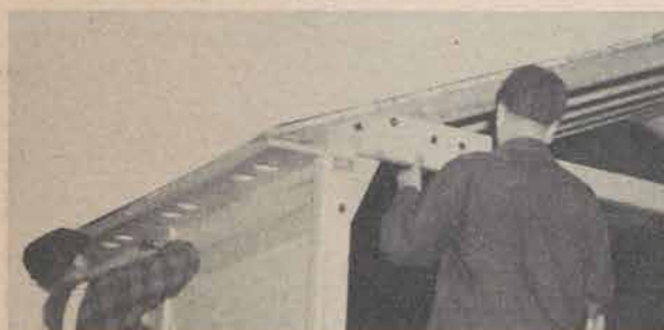
Figure 30. Applying T-4 and eave board.
