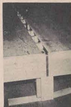
Figure 12. Floor straps in place.
