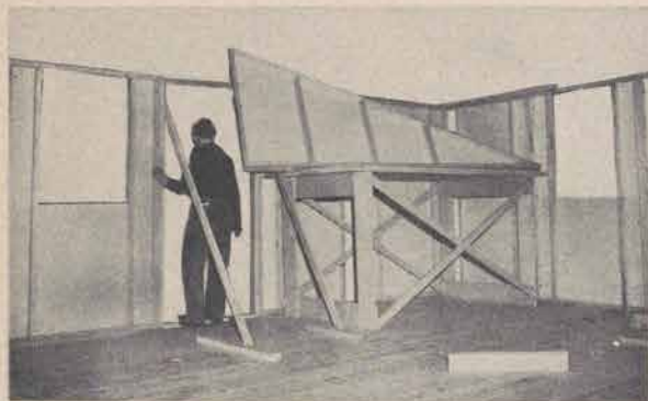
Figure 18. Gable end ready for erection.
