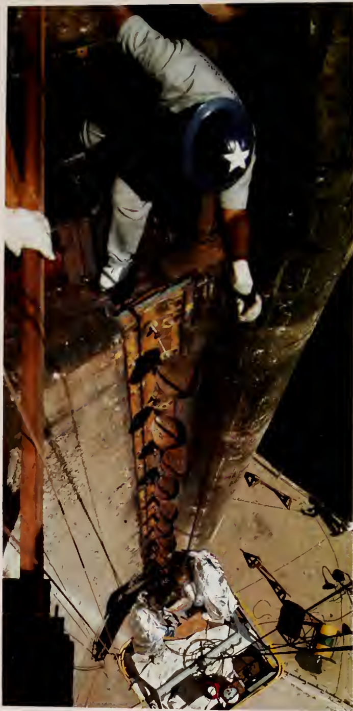
A better way: Left, the pouring of molten babbitt into the hollow quoin bearing platform and faster way to accomplish the task, the juncture at which the miter gate meets the lock wall, was once accomplished by lifting workmen in a basket and lowering containers of babbitt to them. Today the workmen and a container carrying enough of the 650°F metal to complete the whole job are raised at one time on a platform, a brand new 900-pound pintle ball, the lock wall, was once accomplished by which the miter gate rotates, is eased into place, one of the last jobs to be done before the chamber is flooded and the gates are rotated back into position.
