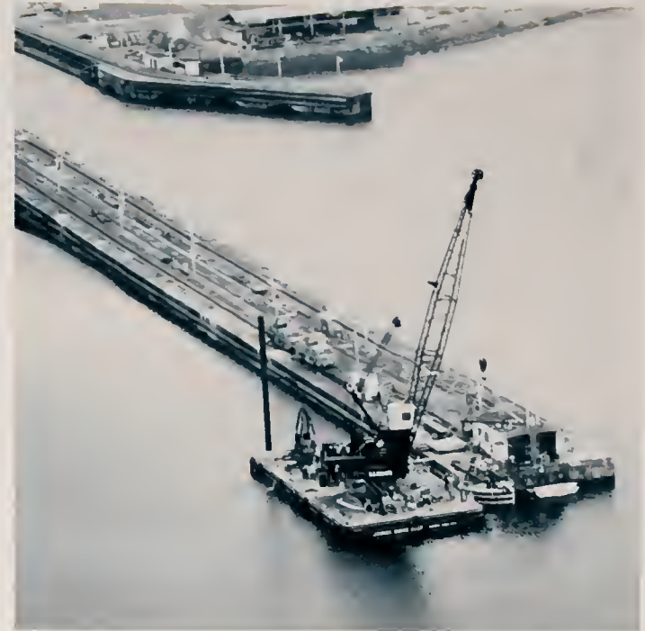
Replacing the softnose at Gatun Locks: Left, at the Maintenance Division shed, employees prepare the wooden form that will hold the concrete for the precast softnose unit. A steel strongback that will check the pressure of the bulging concrete is examined to insure a proper fit, then bolted into place. Center: At high tide the Dredging Division's craneboat "Atlas" lifts the 62-ton unit, one of four pieces of the completed softnose, from Dock 8 to transport it to Gatun. Above: An aerial view of the unit being bolted to the centerwall at Gatun Locks while being supported by the derrick barge "Goliath."
