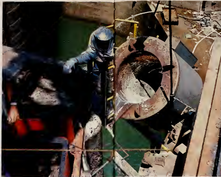
A better way: Left, the pouring of molten babbitt into the hollow quoin bearing platform and faster way to accomplish the task, the juncture at which the miter gate meets the lock wall, was once accomplished by lifting workmen in a basket and lowering containers of babbitt to them. Today the workmen and a container carrying enough of the 650°F metal to complete the whole job are raised at one time on a platform, a brand new 900-pound pintle ball, the lock wall, was once accomplished by which the miter gate rotates, is eased into place, one of the last jobs to be done before the chamber is flooded and the gates are rotated back into position.
