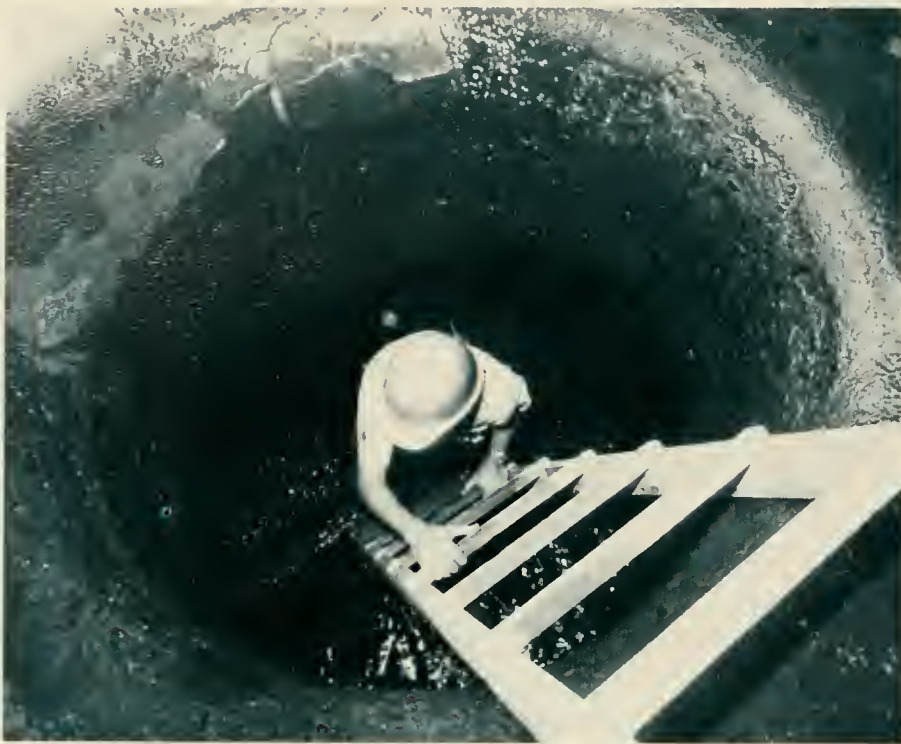
Above: A Locks Division employee descends 8 feet into a 6-foot lateral culvert in the chamber floor to inspect for cracks in the concrete. Below: The mighty miter gates at rest in Balboa Drydock, where they undergo a complete overhaul in a 2-month period. Right, a gate gets a touchup.
