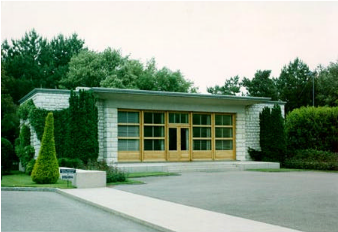
Exterior of the Visitors' Building
