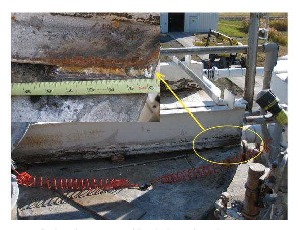
support after the insulation was removed from the slurry tanks 1 and 2. A DuPont engineer wrote up a work order for the repair of the agitator supports and had the construction field engineer in charge of contractors begin writing a work scope and gather contractors and materials. DuPont hired Mollenberg-Betz to repair the agitator support based on the fact that they were already engaged in hot work on site and could be quickly made available.
