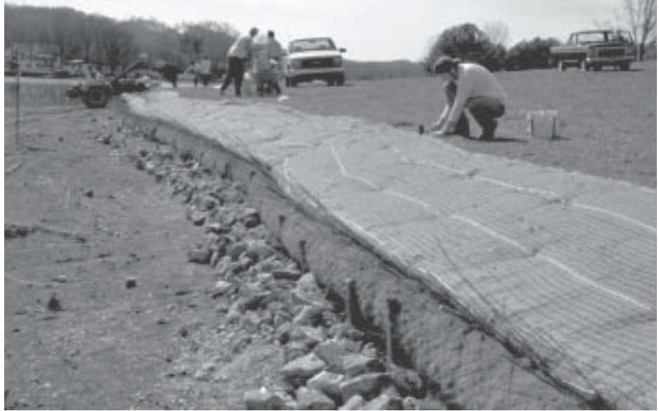
Vegetated Geogrid and Coconut Fiber Roll
