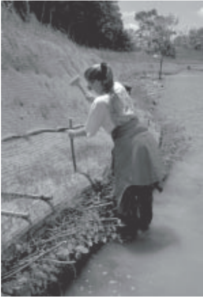
Live Stakes and Coconut Fiber Roll
