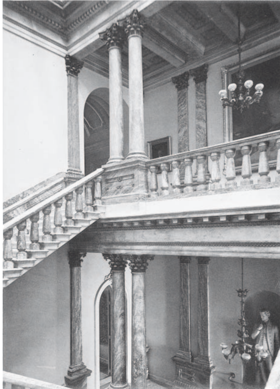
FOUR PRINCIPAL STAIRWAYS, SIMILAR IN DESIGN ON HOUSE AND SENATE WING. This marble staircase is located on the east side of the House wing between the second and third floors.
