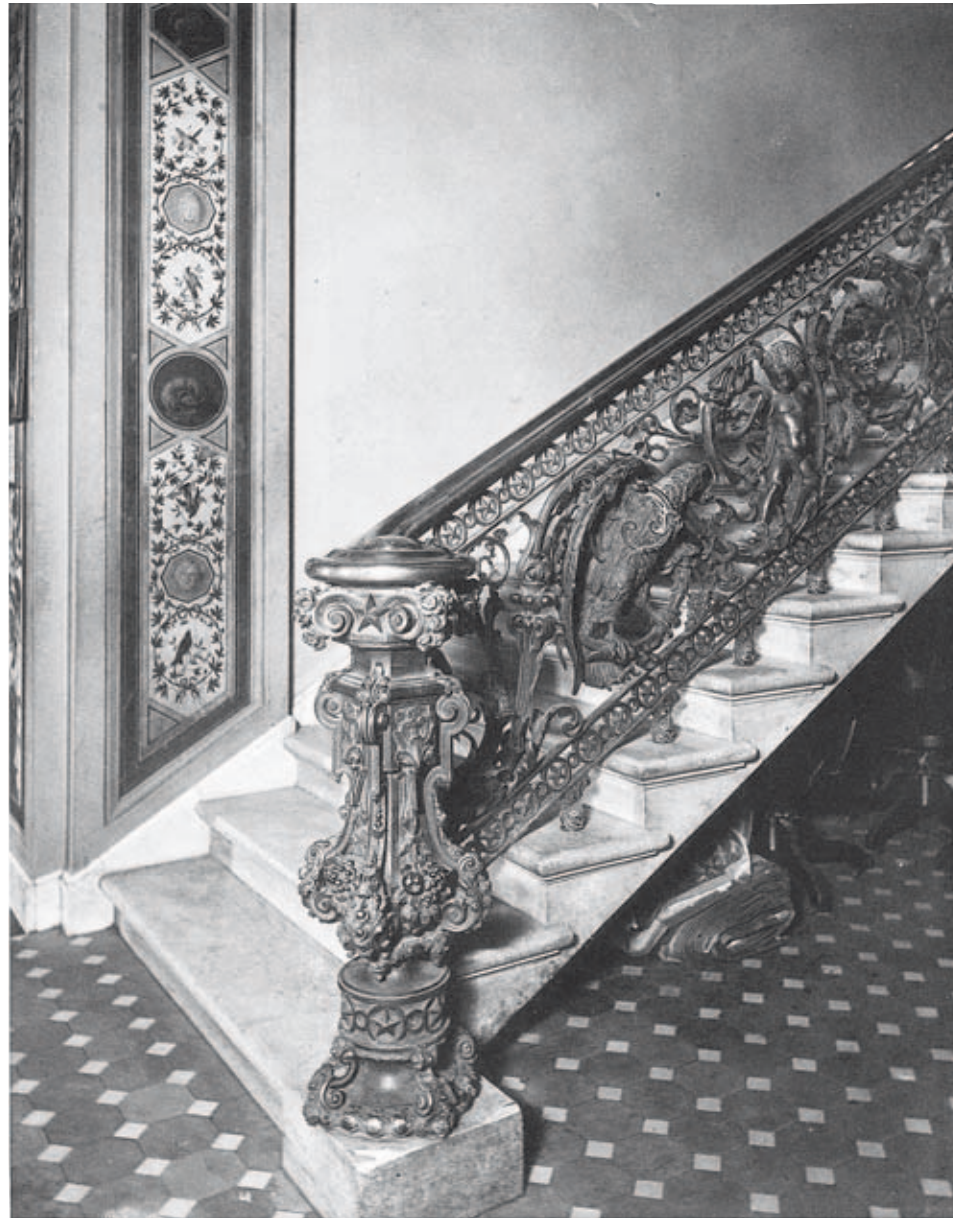
SENATORS PRIVATE BRONZE STAIRWAY, NORTH WING,—T. U. WALTER ARCHITECT. Designed by Constantino Brumidi, modeled by Edmond Baudin, and cast by Archer, Warner, Miskey and Co. of Philadelphia, 1857–59 (related drawing, plate 213).
