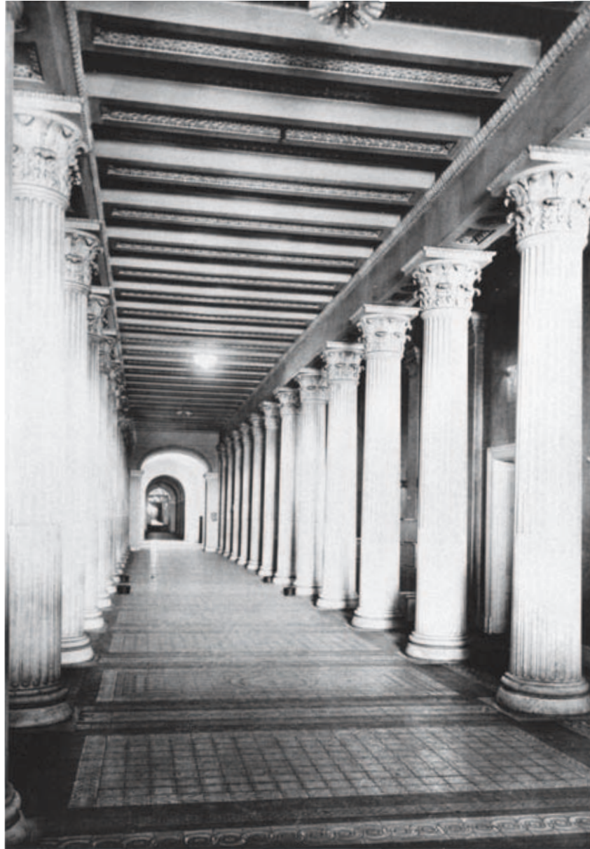
BASEMENT HALL, SOUTH WING.
