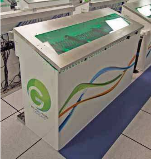
FIGURE 3. The immersion cooling system at the Laboratory for Physical Sciences, like the one pictured above, uses mineral oil to cool IT equipment. (Photo used with permission from Green Revolution Cooling: www.grcooling.com .)
